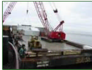
The truck then hauls everything to the barge.
